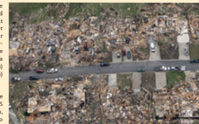
Figure 7-7 Damage in Joplin, Missouri, two days after an EF-5 tornado devastated the city.
